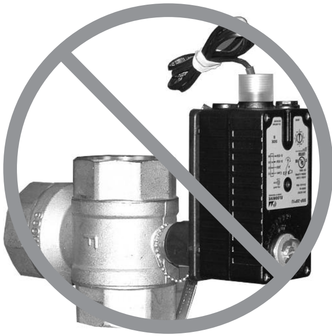
Fig. 20: Incorrect Orientation of Actuator
